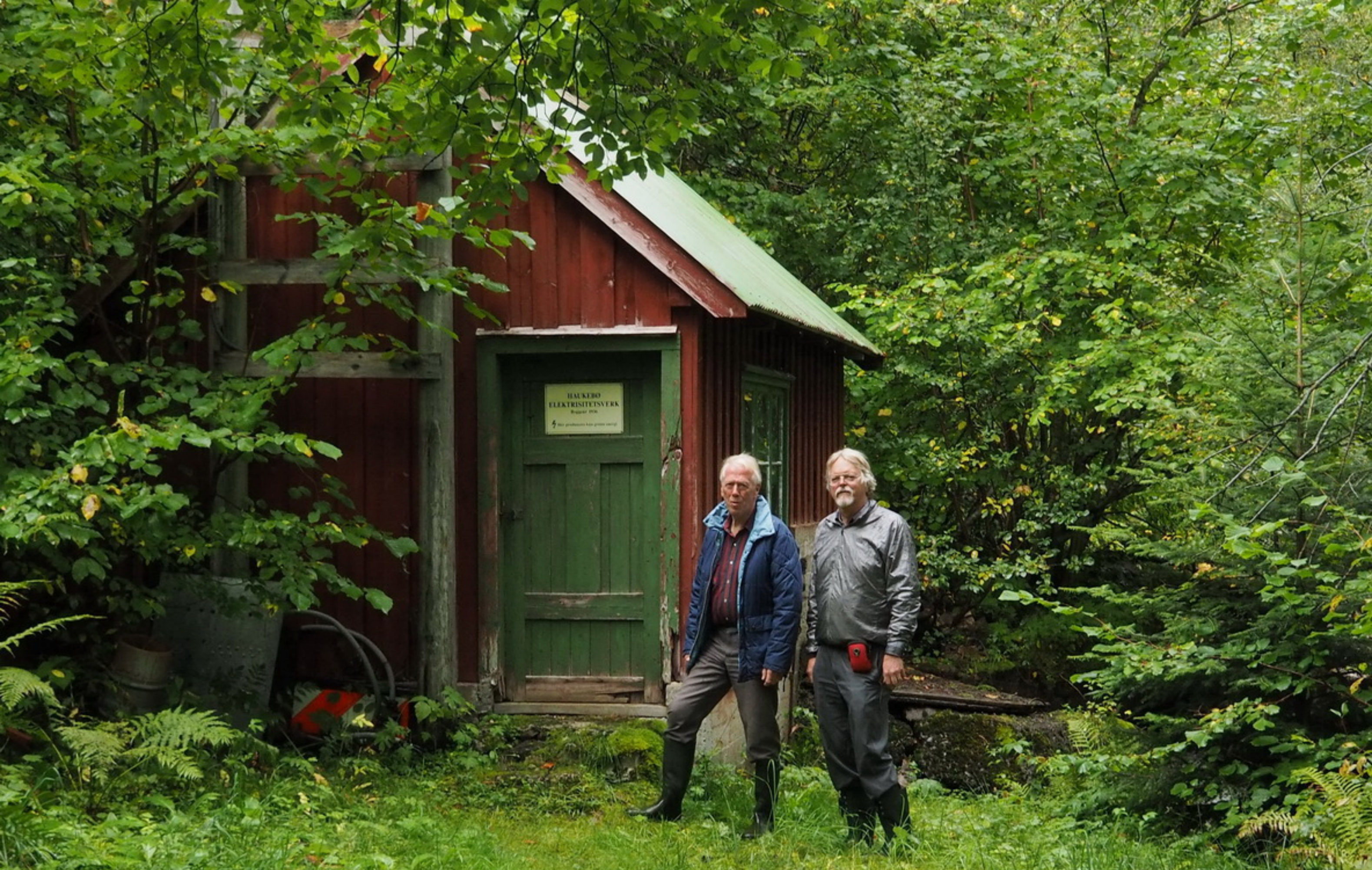
Helge is proud of his historic hydroelectric power plant.
